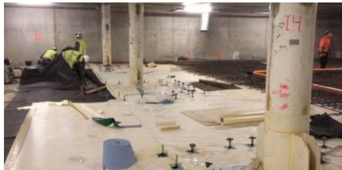
Existing Basements – Box in Box
