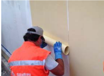
3) Apply membrane in wet adhesive bed
