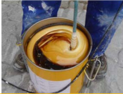
1) Mixing of 2K PU adhesive
