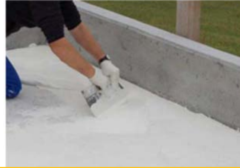
2) Apply adhesive with trowels
