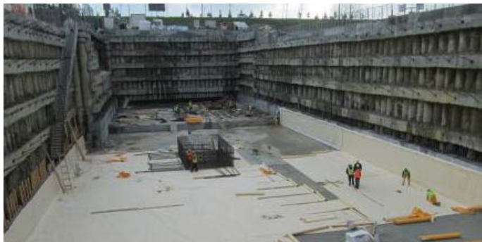
New Basements – Vertical Excavation
