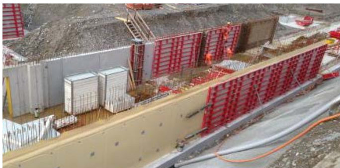
New Basements – Open Excavation
