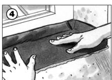
Press on **SikaMembran** sheet using a plastic roller.
